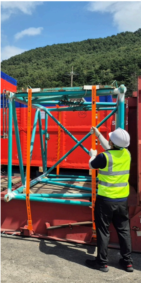
On-site supervision of construction equipment handling.
